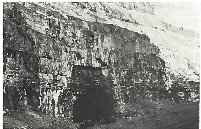
FIGURE 4 Underground mines seldom extracted more than the lower third of the Monarch coal as evidenced by this abandoned portal in the Big Horn No. 1 strip mine near Acme, Wyoming.
