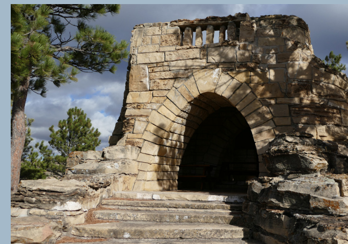
The Castle picnic shelter was built by the Civilian Conservation Corps in the 1930s using sandstone from the Hartville Formation.
