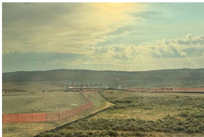
Natrium Facility Build Site Near Kemmerer, WY
