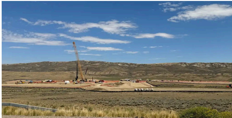
Build site for the Kemmerer Unit 01 Natrium Reactor facility in August 2024.
