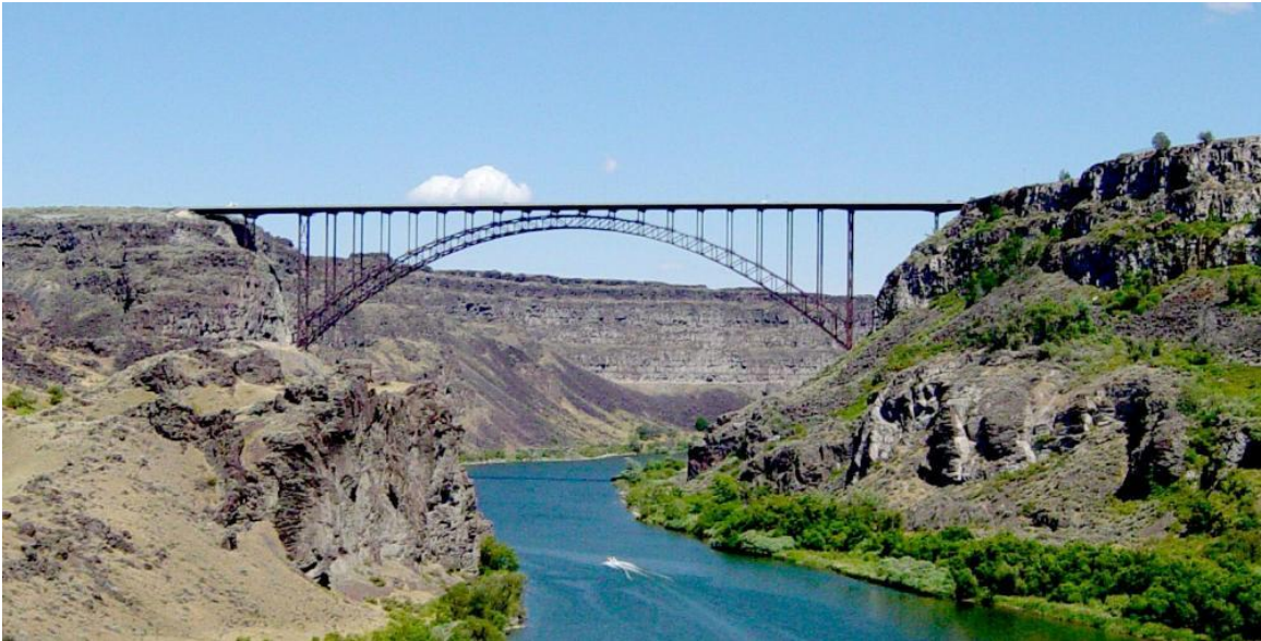
Figure 3: Perrine Bridge at Twin Falls, Idaho.
