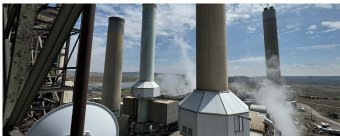
Smokestacks at the Naughton Power Plant.
