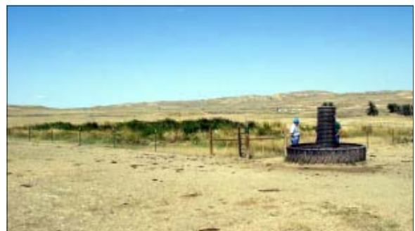
Fig. 7. Constructed wetland (ALL Consulting, 2003)
