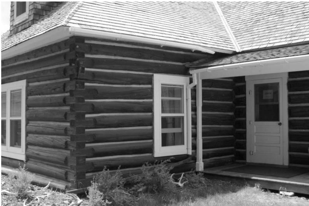
Figure 2. Miller House, view of entrance, east elevation.
