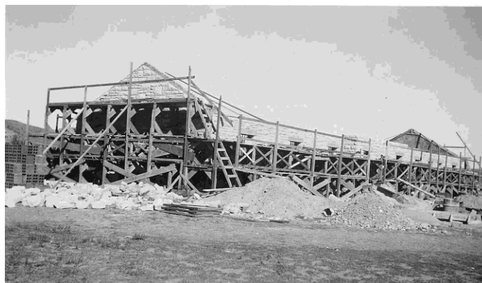
Figure 2 – Construction of Building 101, Oct. 1940 (Meeden)
