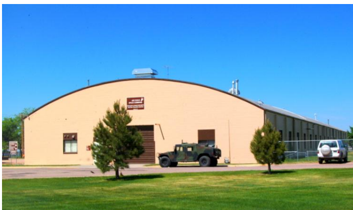
Figure 12 – Building 011, a contributing building in the eligible National Register Historic District
