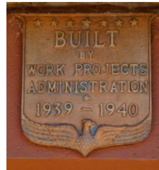
Figure 5 – WPA shield, Building 101
