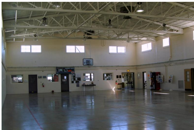
Figure 10 – Drill hall interior, Cody
