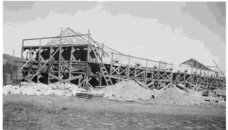
Figure 2 – Construction of Building 101, Oct. 1940 (Meeden)
