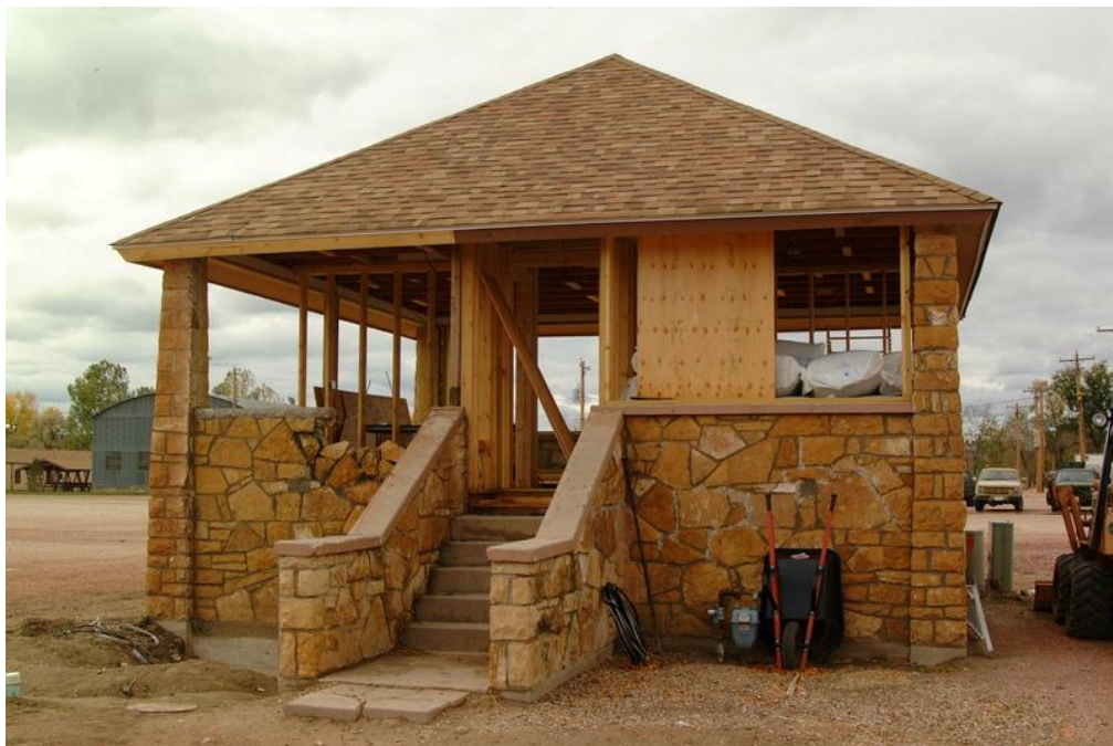
Figure 17– Bandstand (Building 602) undergoing rehabilitation
