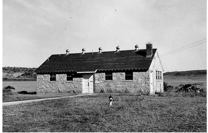
Figure 3– A typical latrine c. 1942 (Meeden)
