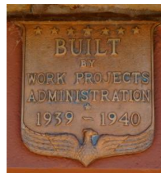
Figure 6— WPA Shield, Building 101
