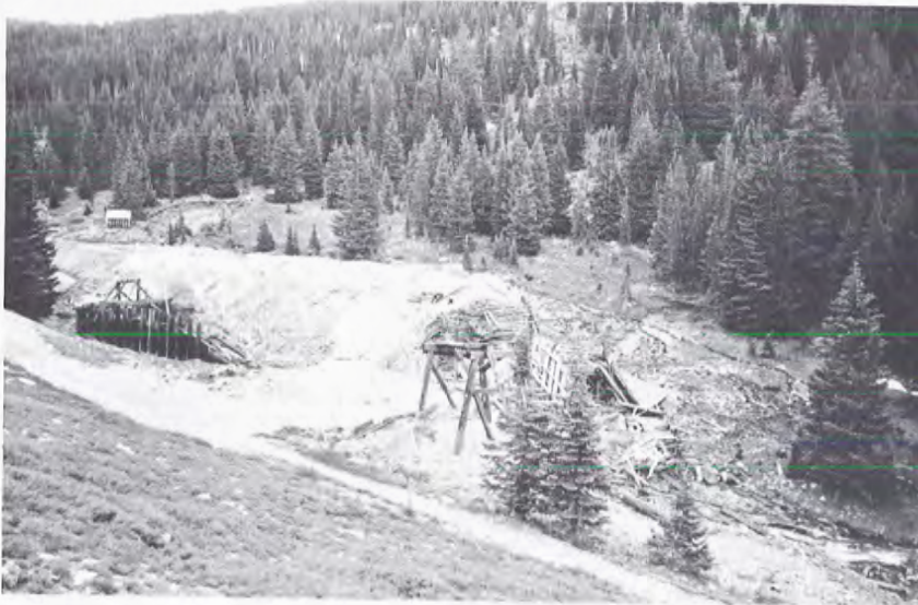
Figure 7. (A) The Ferris-Haggarty mine in 1902. The tramway is located in the right half of the photograph and runs from the mine dump to Encampment 16 miles to the east (photograph courtesy of AHC). (B) The Ferris-Haggarty mine as it appeared in 1983. The same mine dump is located in the photograph with Haggarty Creek seen in the lower right corner. Not much remains of the historic buildings.
